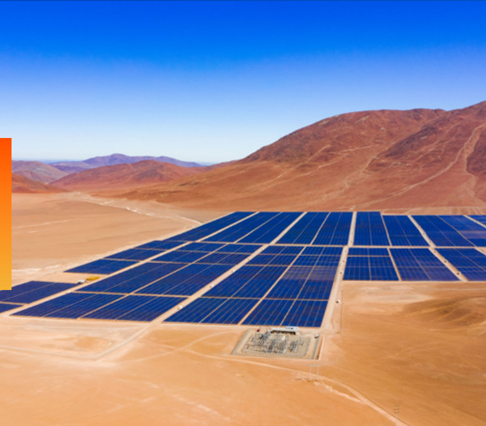
Javiera Solar Plant in Chile's Antofagasta Region
